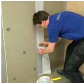
5. Apply self-adhesive fibre glass tape embedded in tile adhesive on the joints (or if necessary waterproofing tape embedded in waterproofing paste).
