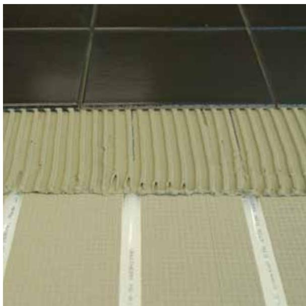
Multiboard is very suitable as insulation for sub floor heating as heating pipe easily can be cut in the boards.
