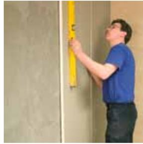
3. Apply the Multiboard against the wall, push and adjust. Then let the adhesive cure completely.
