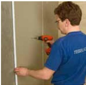
4. Drill through the Multiboard and the cured dabs into the wall and drive in the dowels with 30mm washers.
