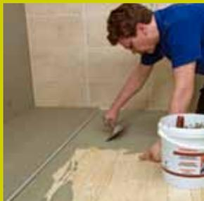
1. Apply on the flat floor Foby PF-Mortar.
