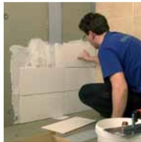
6. Then apply the tiles directly on the Multiboard with tile adhesive.
