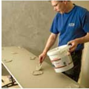
2. Apply 8 dabs of Foby PF-Mortar of at least 2 cm thickness on the holes in the Multiboard.
